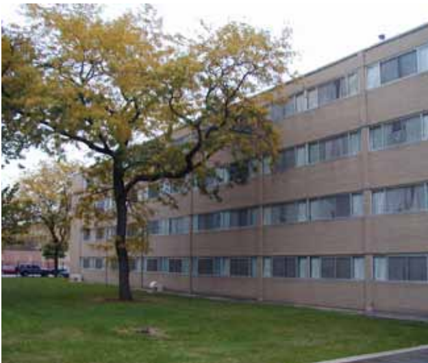
McCormick Student Residence
